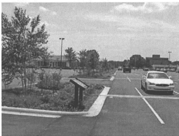
FIGURE 5-27 North Carolina Retrofit Bioretention SCMs. SOURCE: Traver.
